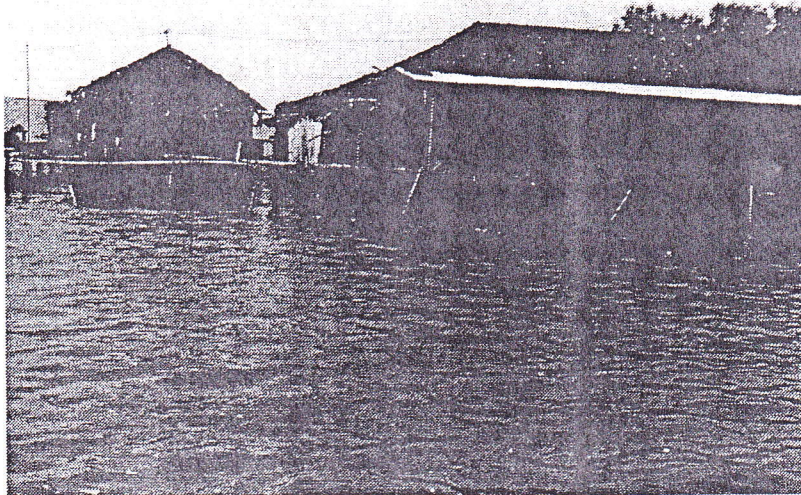
Figure 4: House Stage: increasing elevation of the floor in the village Bedono
